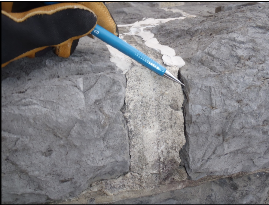
Photograph 3 – Cracked Mortar
