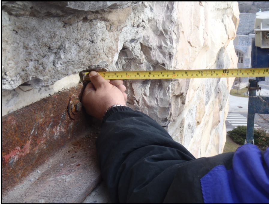
Photograph 2 – Opening in Hokie Stone to Inspect Concealed Conditions
