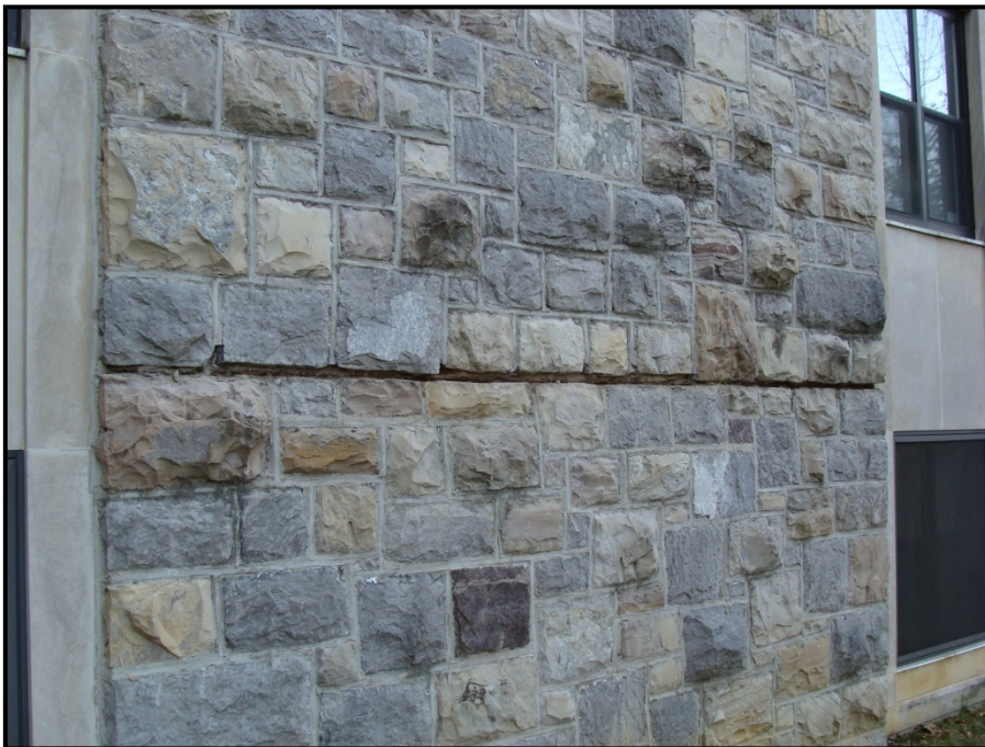
Photograph 5 – Failed Flashing at Shelf Angle
