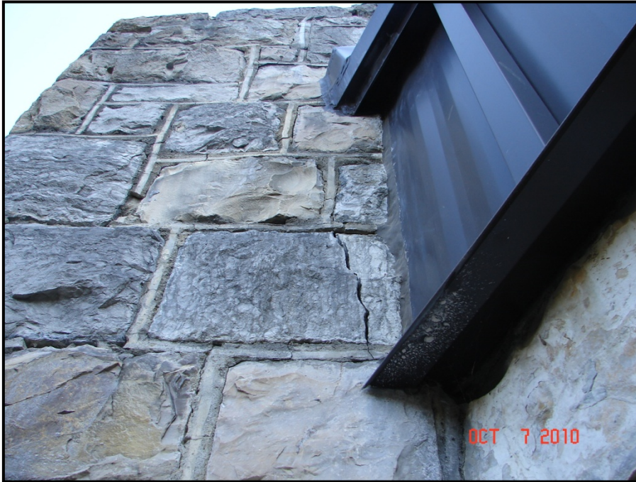
Photograph 4 – Cracked Stone
